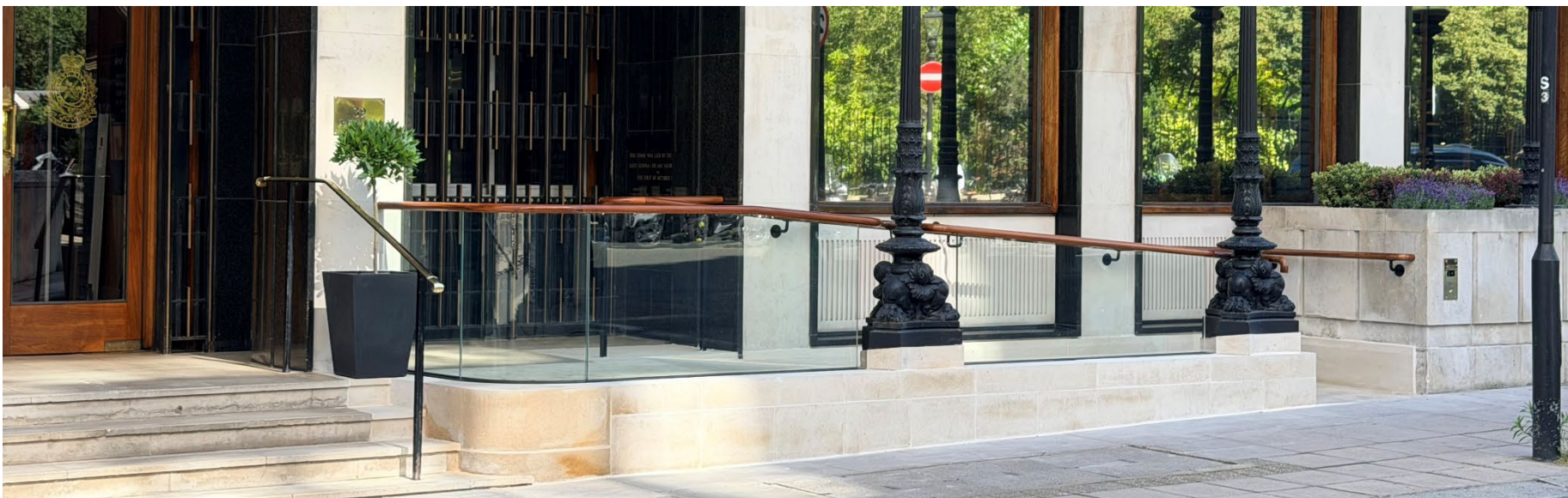
THE ACCESSIBILITY RAMP
